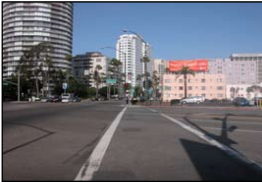
View 4: Looking west at Ocean Boulevard at existing high-rise residential uses south of the project site.
